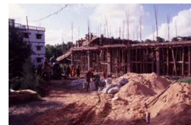
Top: The main schoolhouse and girl's dormitory. Above/Center: The new boy's hostel Left: New staff quarter building
